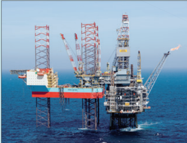
The drilling rig "Maersk Inspirer"
