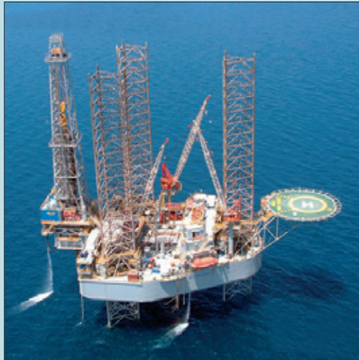
The drilling rig, "Jimmy Puckett", Noble Corporation
