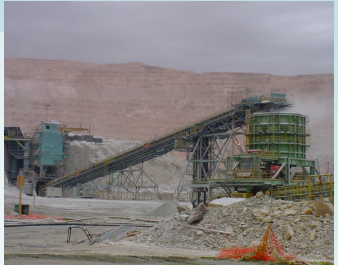
BHP Minera Escondida site in Chile
