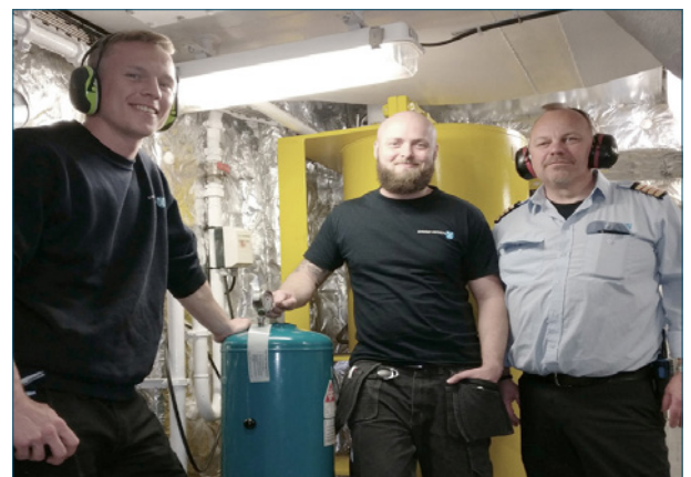
A happy crew next to the CJC® Lube Oil Filter, which replaced a Centrifuge Separator
