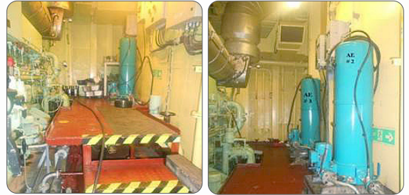
Installed CJC® Oil Care Systems 27/108
